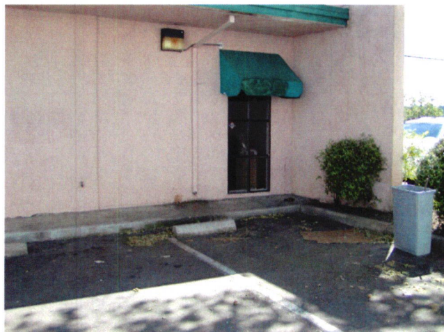
10131 Folsom Blvd (West Side of Building After)
