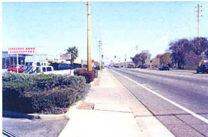
New Concrete Poles to Replace Existing - Relocated on Southside
