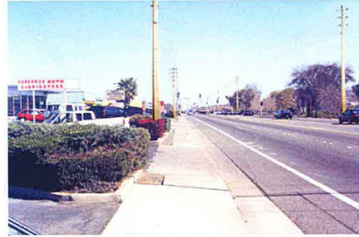
New Concrete Poles to Replace Existing
