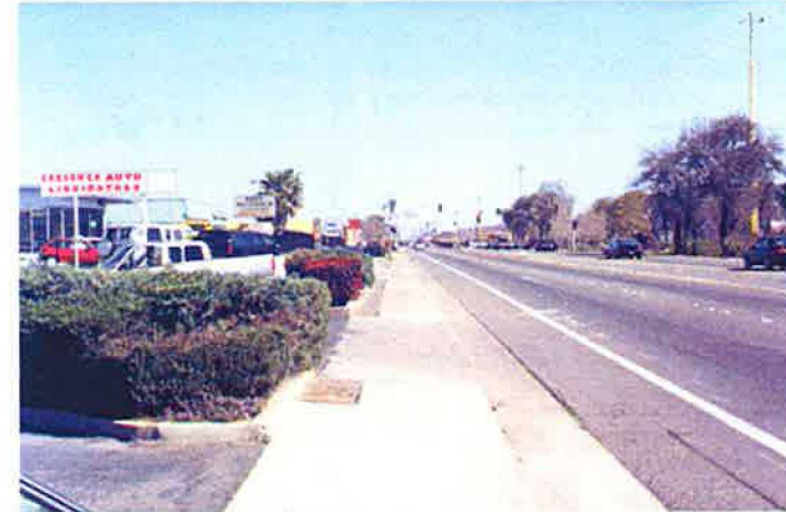
New Concrete Poles - Underground Utilities (Telecom & 12KV)
