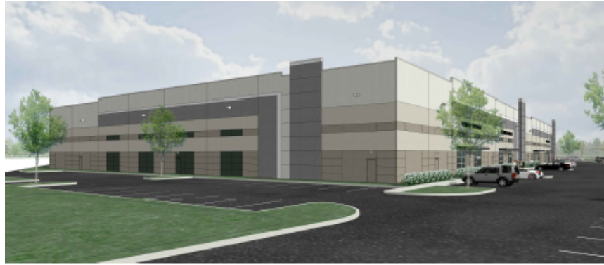
C: VIEW FROM THE NORTHEAST CORNER LOOKING WEST
